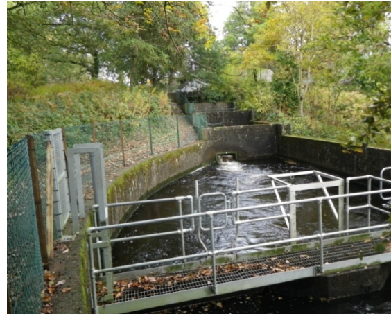
Plate 1d: Resting pool 3 showing central weir with submerged orifice and Vaki fish counter with PIT detector 8 in the background
