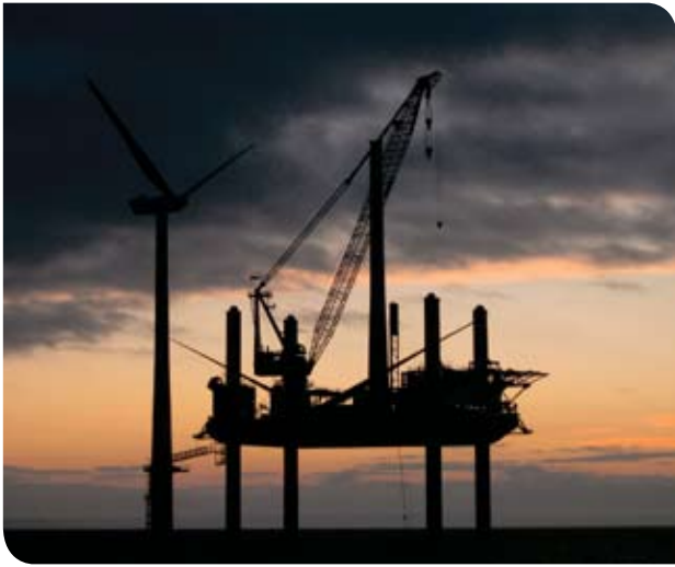
FIRST COMPLETED TURBINE INSTALLATION AT ROBIN RIGG
