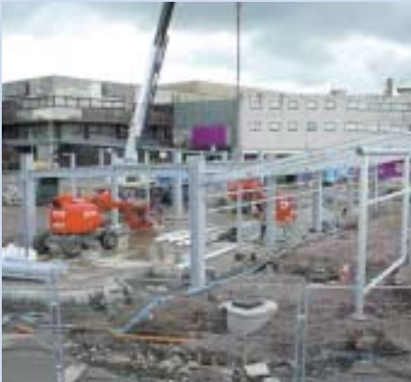
Re-building of East Kilbride Bus Station
